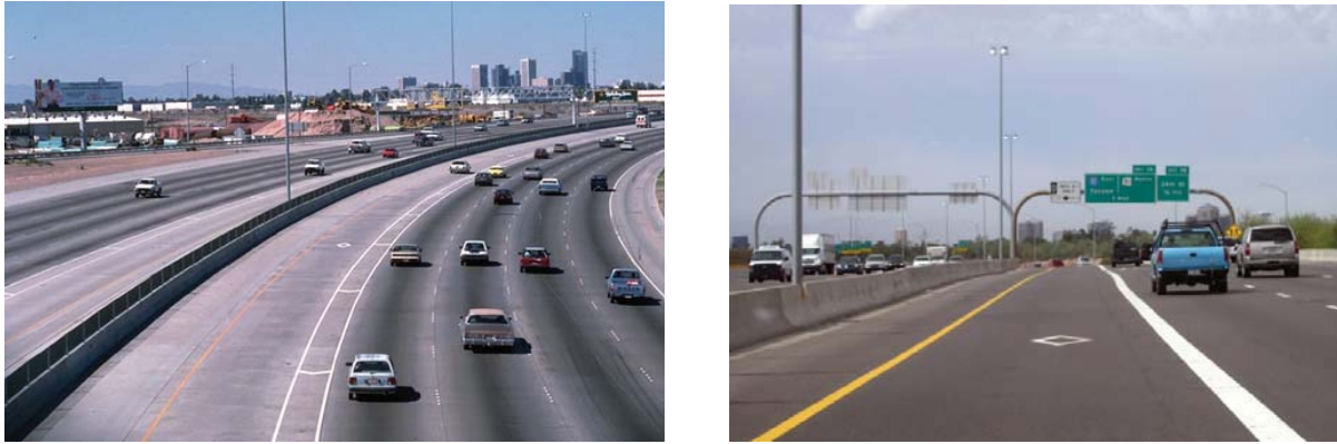
Figure 3-1 Sample Lane Separation Treatments on Phoenix-area HOV Lanes
