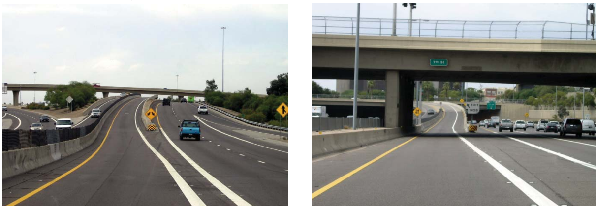
Figure 3-2 Sample DHOV Ramps in the Phoenix-area
