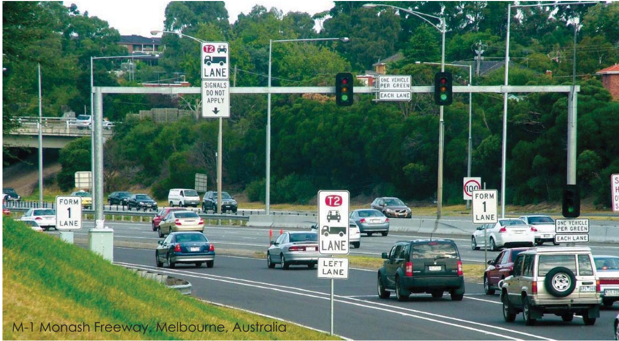
Figure 8-2 Example Managed Freeway
